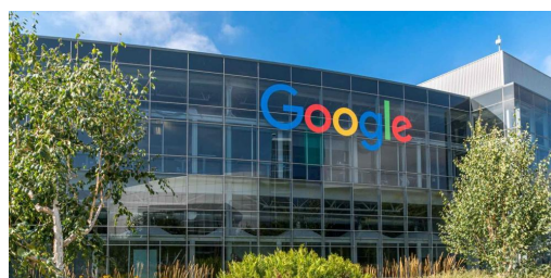
Google Data Center 3.4 Miles
